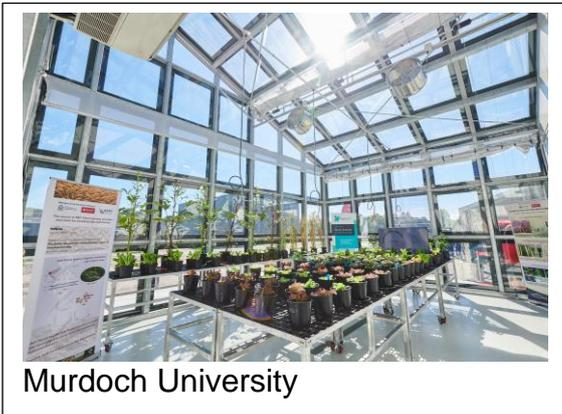
ClearVue’s patented innovative glazing technology uses an activated interlayer, sandwiched within a panel composed of a number of glass panes, some of which are coated by specialised thin-films. Our advanced glazing system combines: our proprietary nano and micro particles dispersed into an interlayer; a clever internal design; and our custom shaped PV cells.
